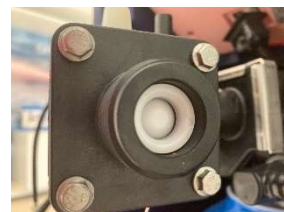
Softener head connection flange (IN/OUT)
